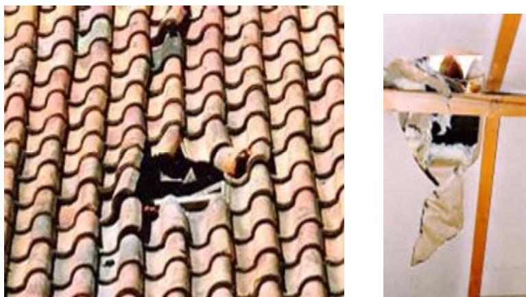
FIGURE 4-15 Damage to a tile roof and the interior ceiling caused by the strike of a meteorite of estimated mass 0.7 kg with an impact speed of less than 500 ft/s, illustrating the limited damage potential of kinetic energy warheads. Increased speed of impact on structural elements such as walls and roofs does not cause proportional increases in lateral damage, but primarily increases the number of walls and such that can be penetrated.
