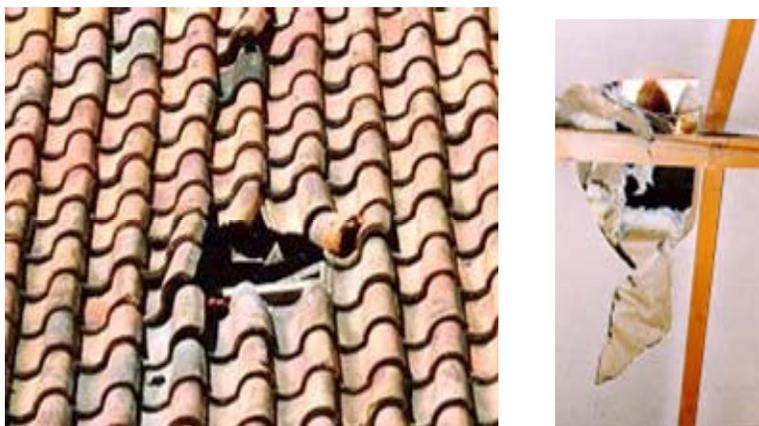
FIGURE 4-15 Damage to a tile roof and the interior ceiling caused by the strike of a meteorite of estimated mass 0.7 kg with an impact speed of less than 500 ft/s, illustrating the limited damage potential of kinetic energy warheads. Increased speed of impact on structural elements such as walls and roofs does not cause proportional increases in lateral damage, but primarily increases the number of walls and such that can be penetrated.
